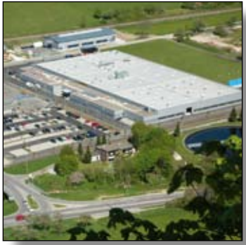
New plant 2 in Albstadt: Investment for PCD production
