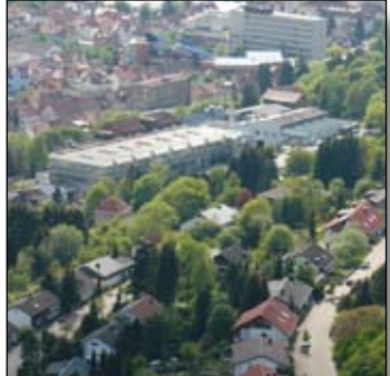
Guhring headquarters: Plant 1 in Albstadt.
